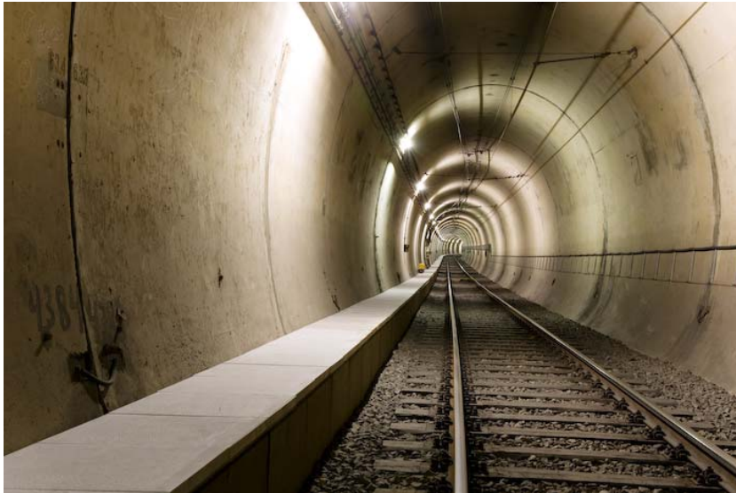
Bored Tunnel Example
